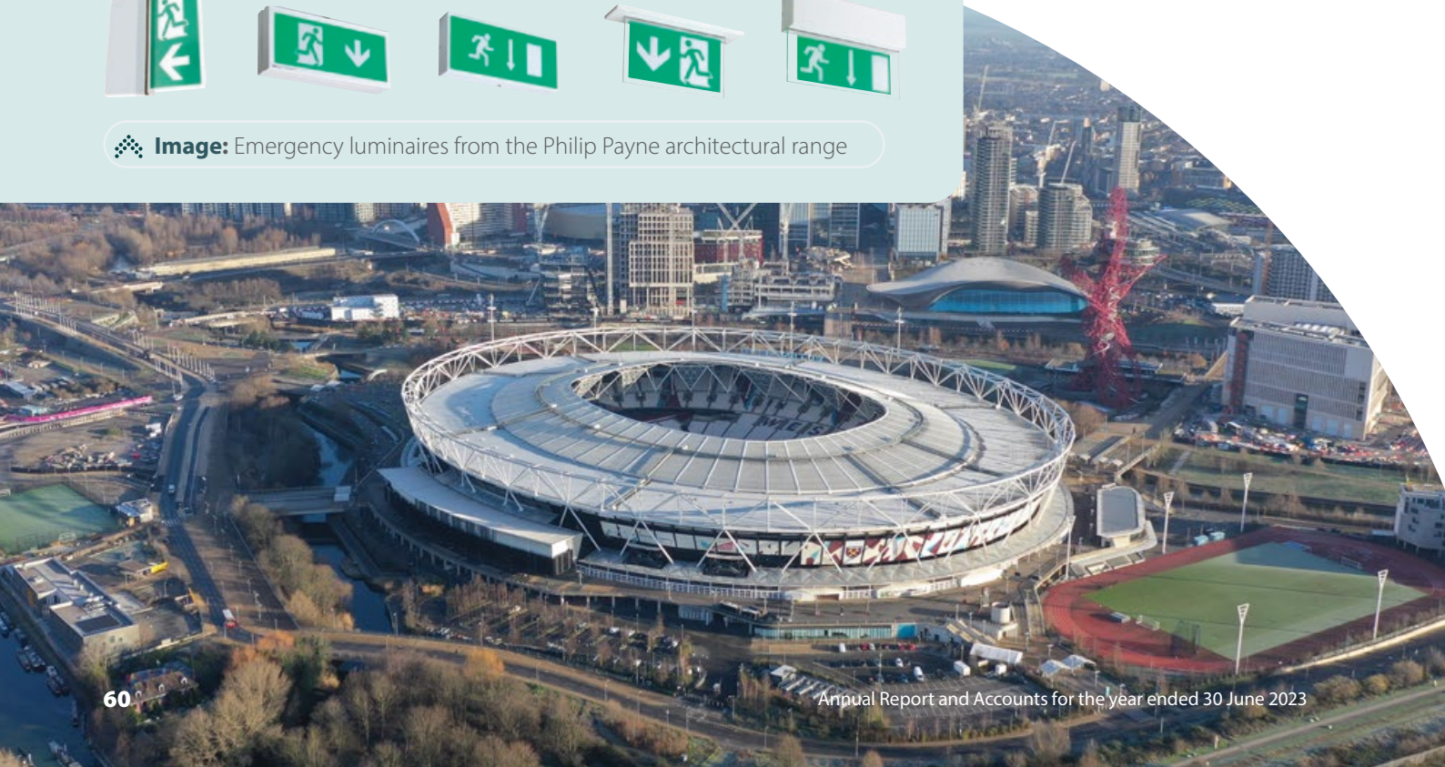
Image: Philip Payne secures the retro fit exit signs for London Stadium
